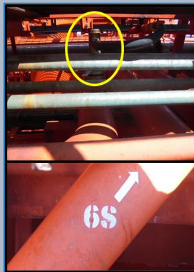
Pressure sensor under the catwalk and stencil with an arrow indicating the location of the pressure sensor
